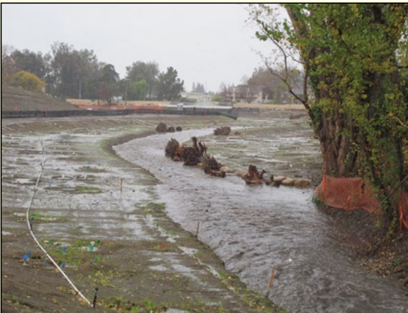
Balance Hydrologics restoration project on Penitencia Creek
